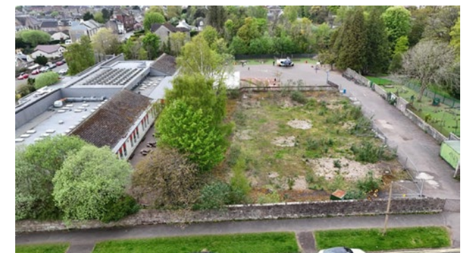
Aerial view of the Annex Site at Hermitage Primary School
