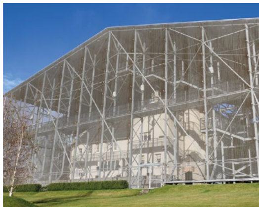
The Hill House, inside its protective 'Box'
