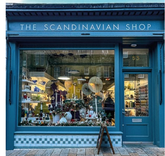
The Scandinavian Shop, an example of a traditional Helensburgh shopfront restored with CARS funding
